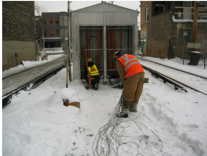
Cable Installation Francisco Relay House
