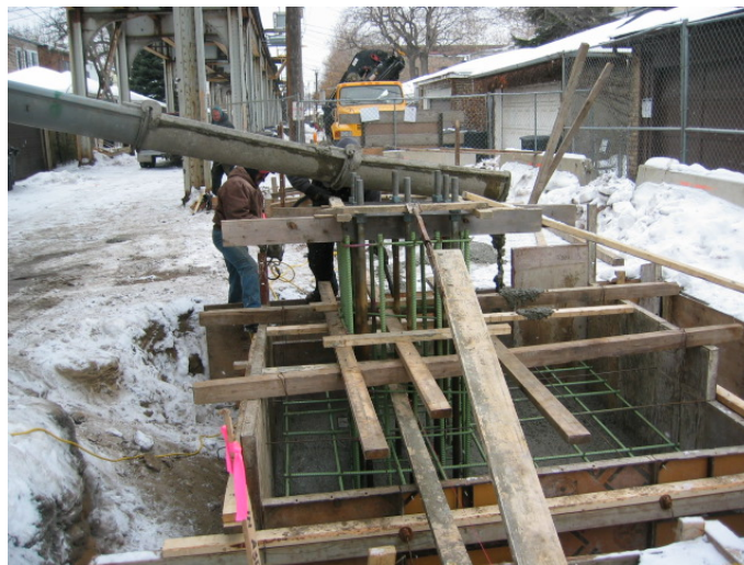
Relay House Foundation Installation at Lake and Seminary
