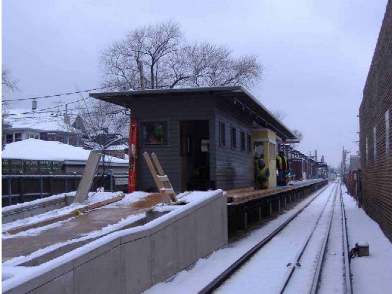
Installation of Francisco station house
